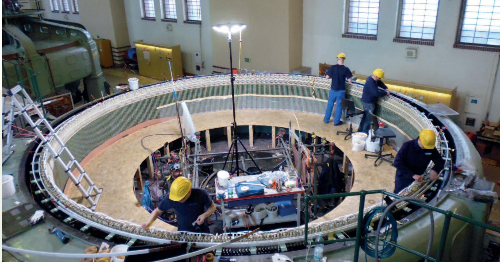
Assembly of coils on-site. The service technician stands in the 7000 mm wide groove of the stator
