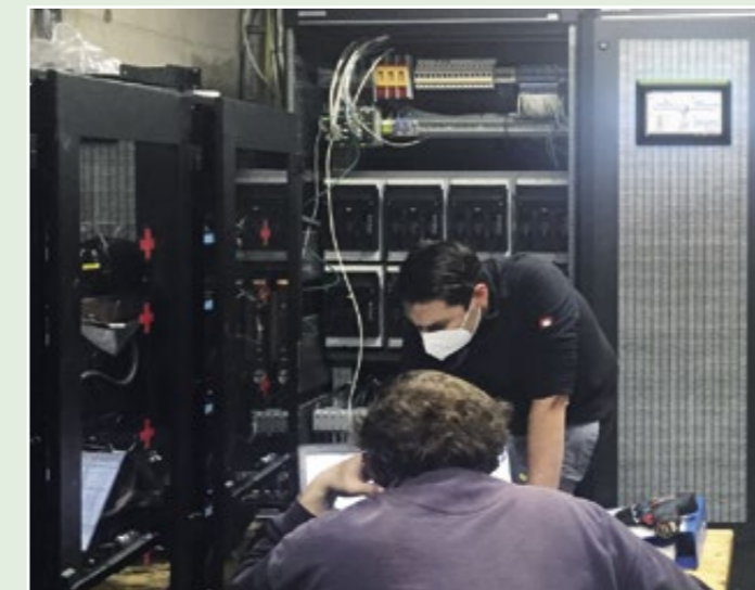
Smart networking of a pre-existing type S7 EMS with the new components.
