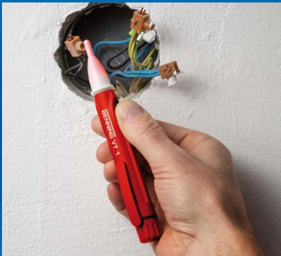
Phase test in junction boxes with BENNING VT 1
