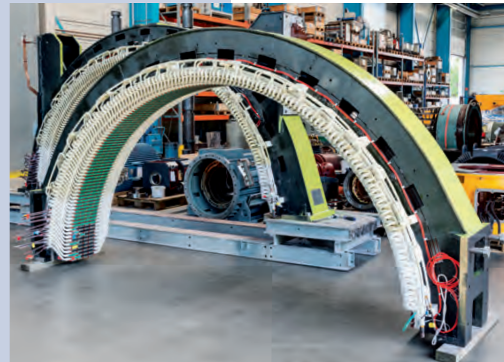
The reconditioned segments before being transported back to the Lech River
