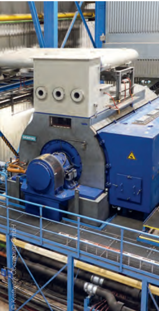
Generator part of the 60 MW gas turbine
