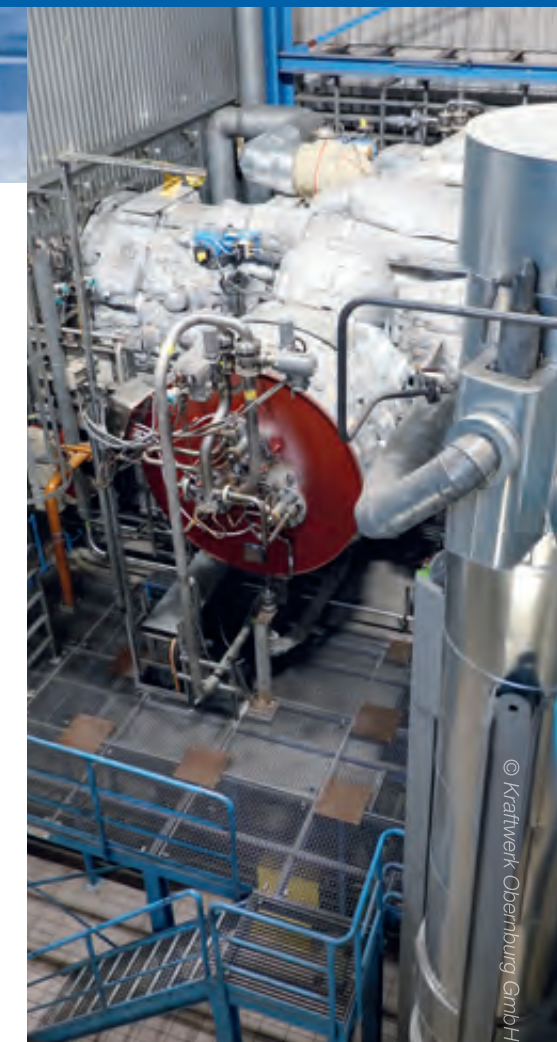
The fuel supply at the gas turbine in the area of the turbine rotor
