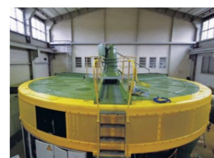
Generator following completion of re-installation at Harbach run-of-river power station
