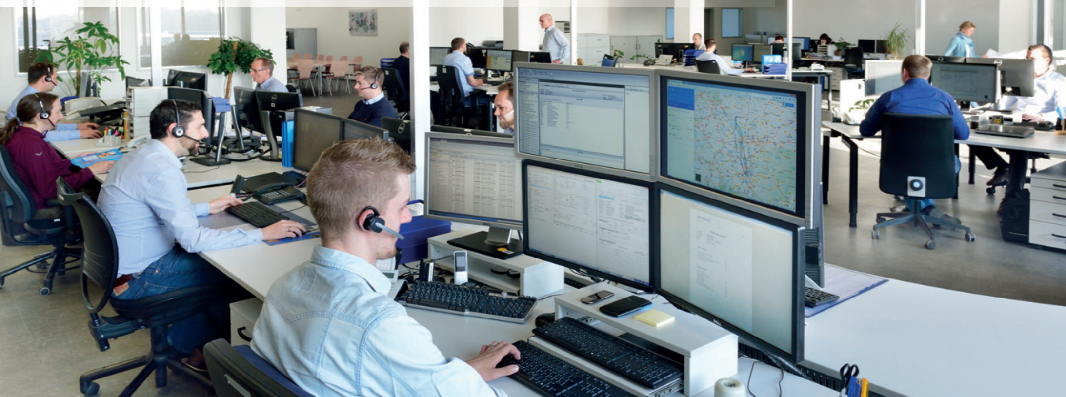
Your power supply system can be monitored continuously and controlled preventively via remote access.
